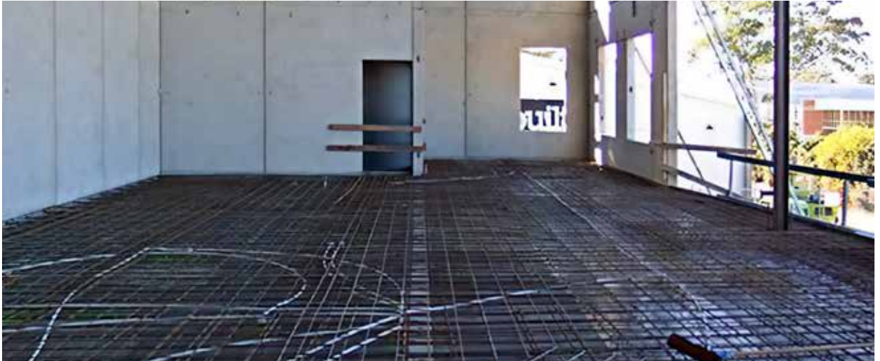
Figure 9.7 Insitu floor and precast wall
