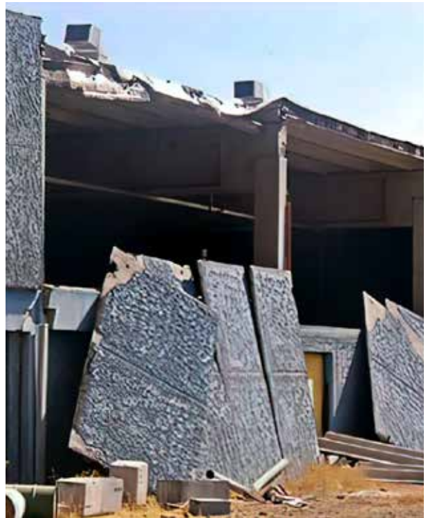
Figure 2.7 In-plane failure of cladding panel connections
