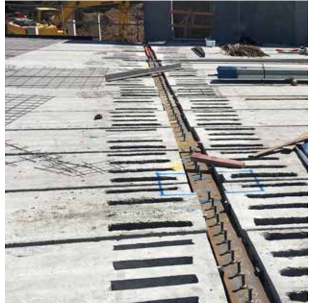
Figure 9.3 Composite steel beams and hollowcore floor
