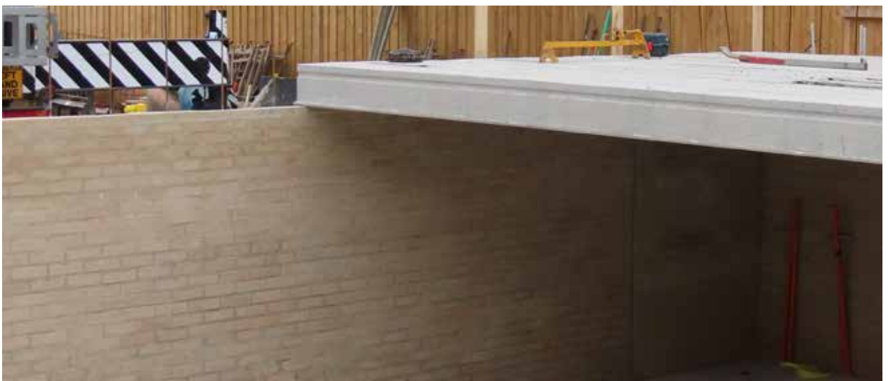
Figure 9.11 Masonry wall and precast floors
