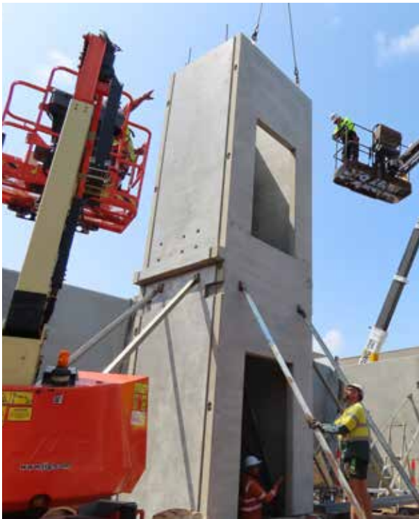
Figure 4.2 Example of precast core with multi-level panels
