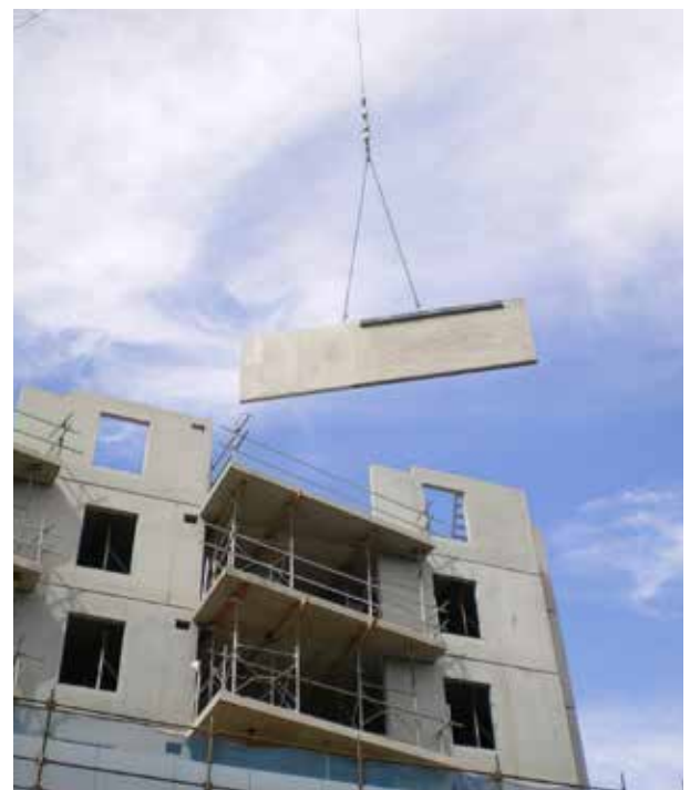
Figure 3.11 Apartment buildings with loadbearing and shear walls
