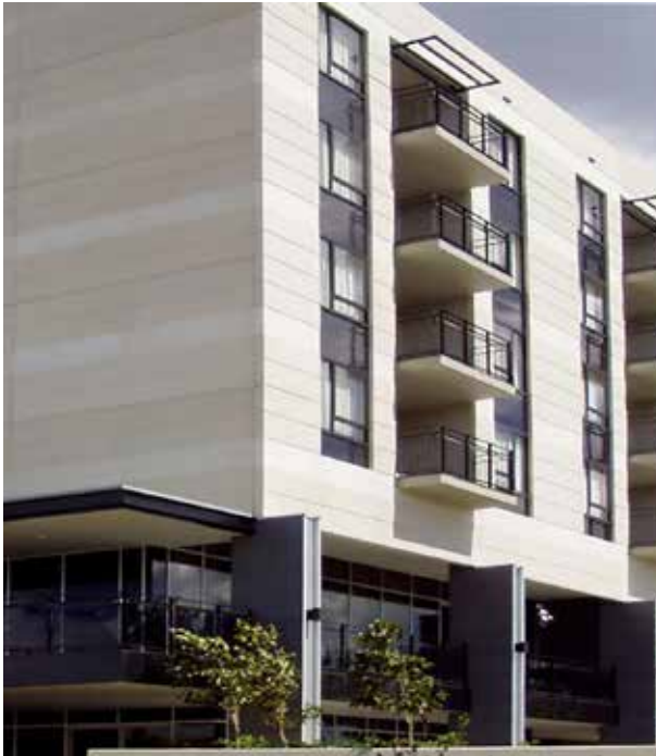
Figure 3.13 Hotel building with open lower levels and loadbearing upper levels
