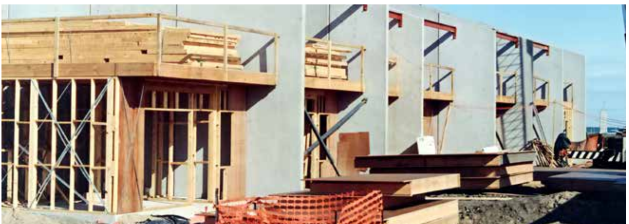
Figure 3.10 Hybrid construction, steel frame roof, timber floors and precast walls
