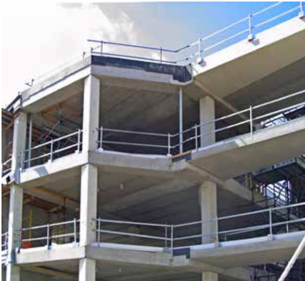
Figure 4.9 Precast columns in frame structure
