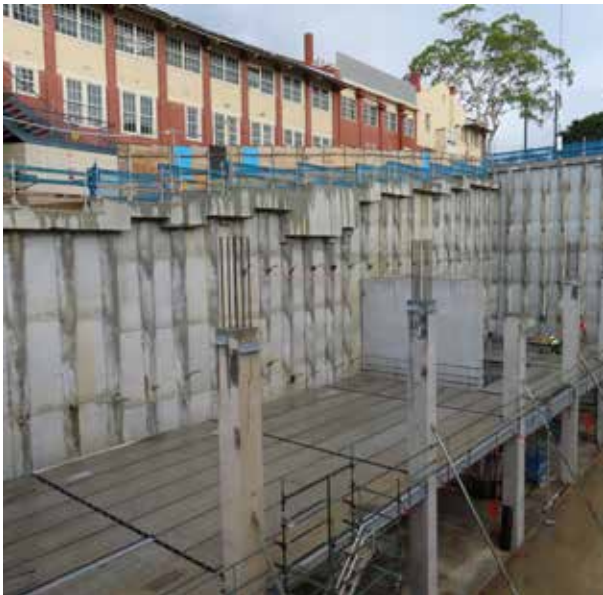
Figure 3.15 Educational building & auditorium
