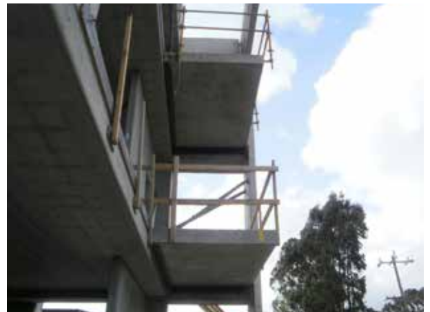
Figure 3.7 High-rise apartment building with loadbearing walls and precast floors
