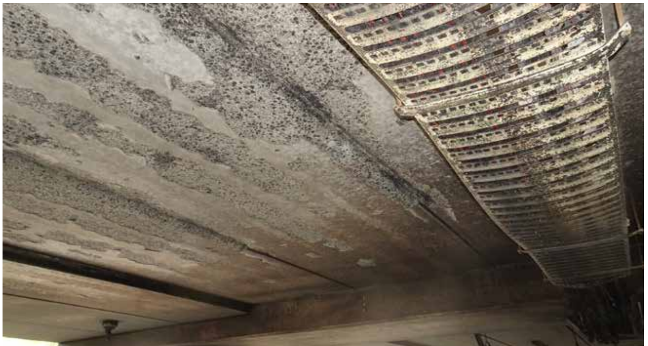
Figure 10.3 Example of heat damaged concrete
