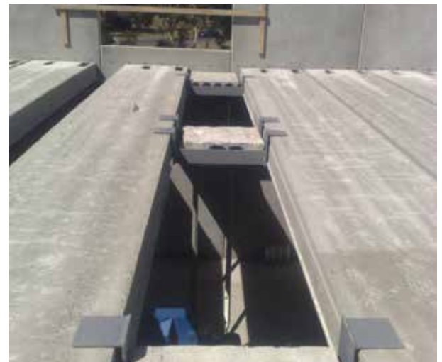
Figure 4.27 Use of trimmer angles or beams for large voids
