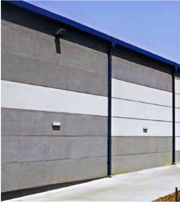
Figure 3.1 Horizontal cladding structure
