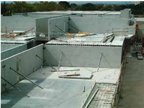
Figure 3.6 Low-rise apartment building with load-bearing cross-walls and corridor walls
