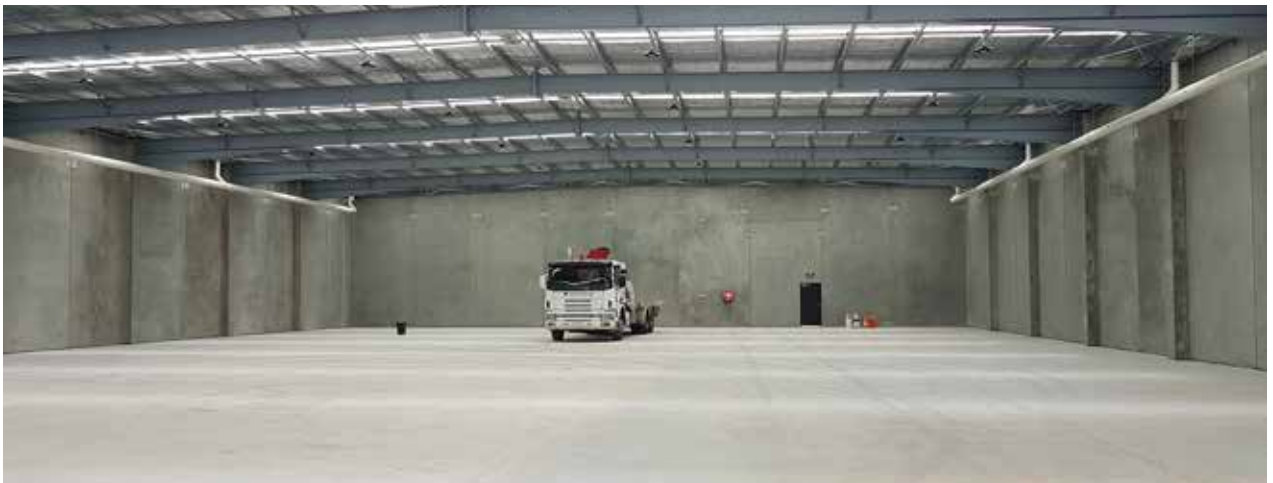
Figure 3.16 Example of braced wall system on industrial building
