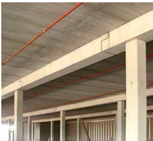
Figure 7.12 Inverted-tee beams designed with a dapped joint to create a negative bending moment at the column that will reduce the depth of the beam
