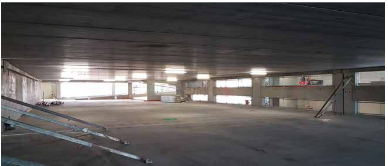
Figure 3.8 Load-bearing facades and clear-span floors
