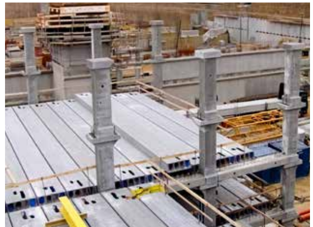
Figure 4.10 Multi-level columns with corbels
