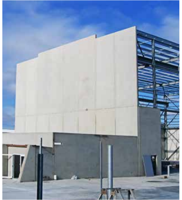
Figure 3.2 Braced wall structures
