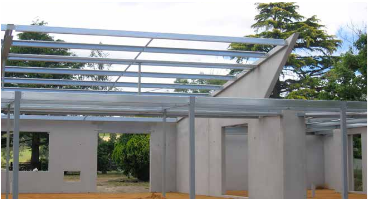
Figure 3.3 Braced wall structure for residential building
