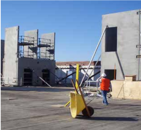
Figure 5.6 Example of precast central cores
