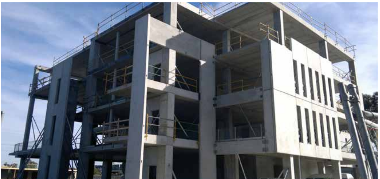
Figure 8.4 Commercial building with multi-level loadbearing walls
