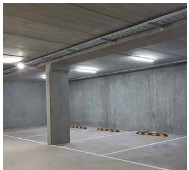
Figure 5.9 Example of precast concrete shear walls
