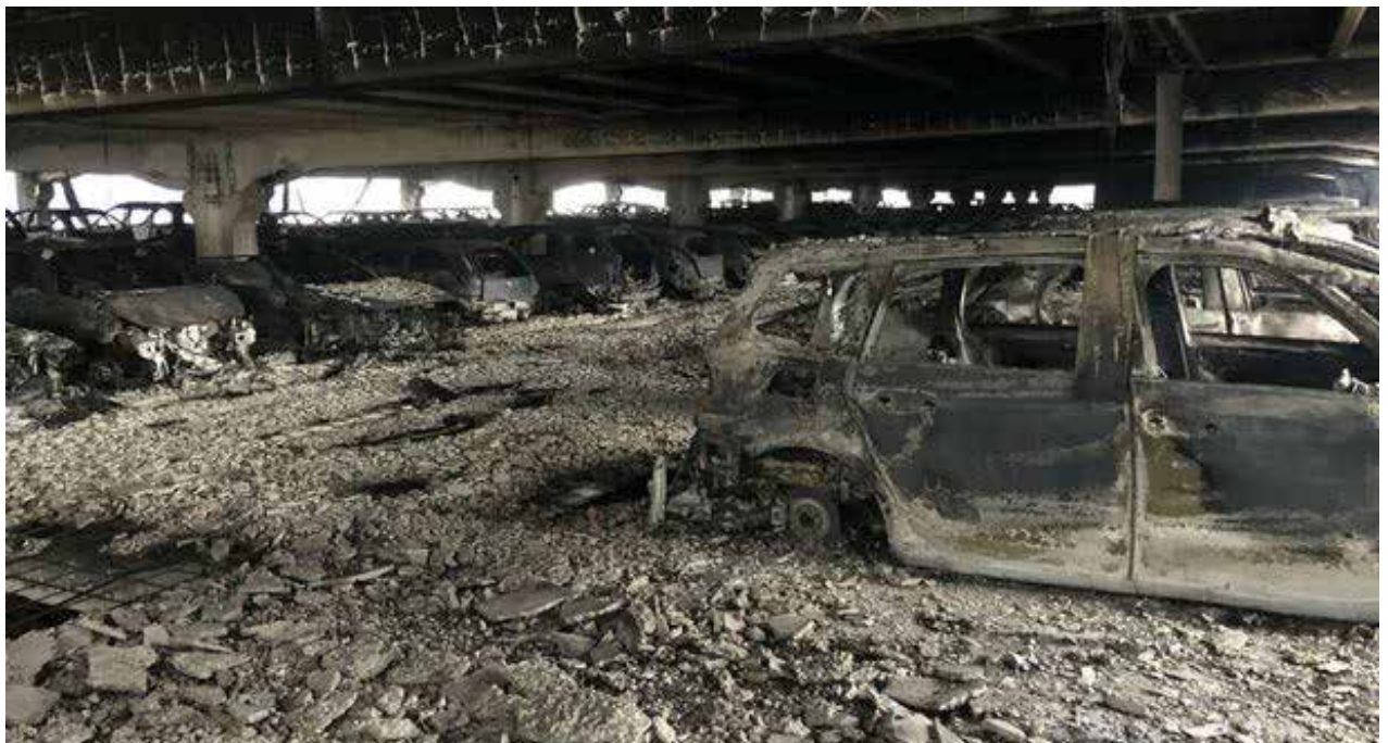
Figure 10.2 Example of a fire damaged car park
