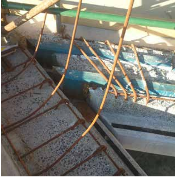
Figure 7.19 High capacity steel hanger brackets
