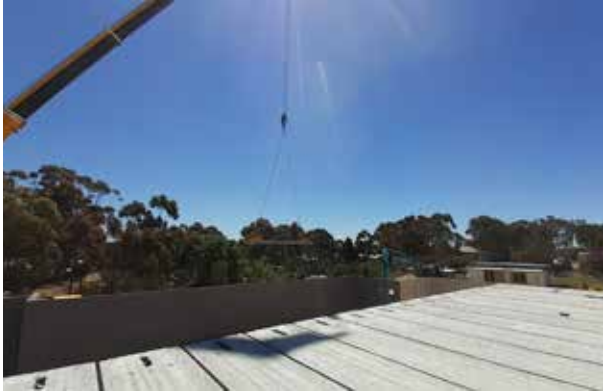
Figure 4.23 Hollowcore floor
