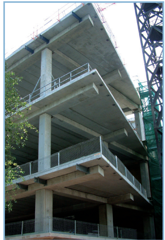
The striking North West corner of the new GPO structure at the corner of Elizabeth Street and Little Bourke Street. Note the requirement of a cantilevered floor in two directions.
