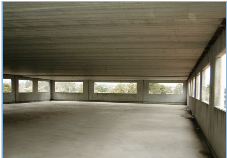
Spans up to 17m give clear, uncluttered space.
