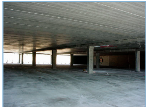
Precast columns and beams used to complement the long span Hollow Core planks.
