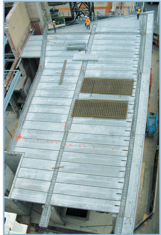
Typical footprint of the GPO structure during construction.
